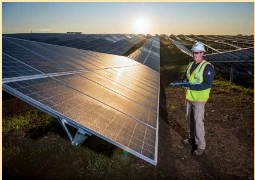
Bill Gatherwright checks one of the 32,000 panels in Cooperative Solar Farm One, which was built last year by East Kentucky Power Cooperative. Photo: Tim Webb
